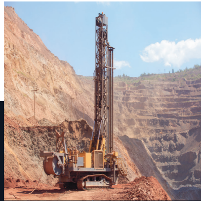
DRILL AND BLAST
